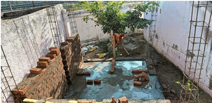
Toilet Under Construction at Nani Silod
